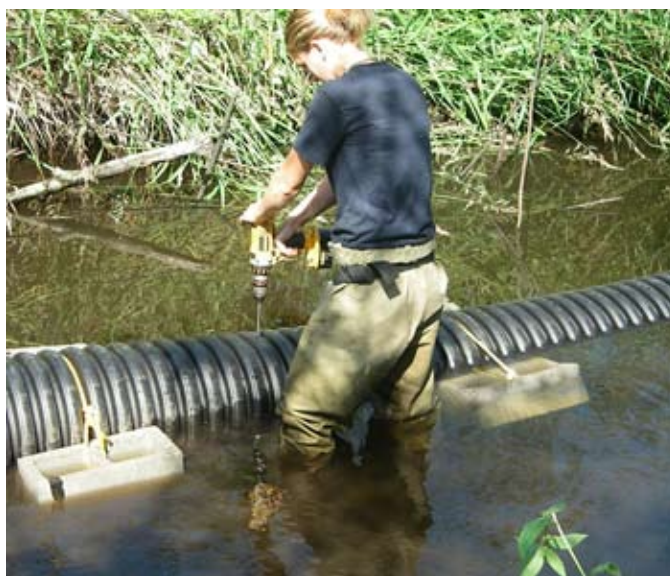
Drilling holes in a flex pipe allows air to escape so it sinks.
