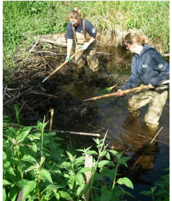
Two interns make a notch in a dam for a flex pipe.
